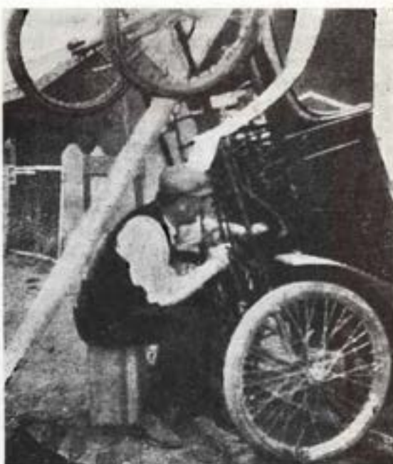
A Scorched Boiler. Expanding the Tubes at Peria.
