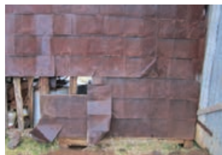
Opened up petrol tins used as farm shed cladding.
