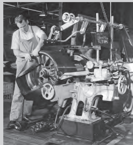
Gordon Harker is turning down the edge of the first 'pocket' of a tyre; then a bead assembly will be fitted, and the fabric turned up to cover it; on a typical truck tyre there would be a second pocket and bead, then a final pocket, and finally the tread and sidewall. Photo uhcl.recollect.co.nz
