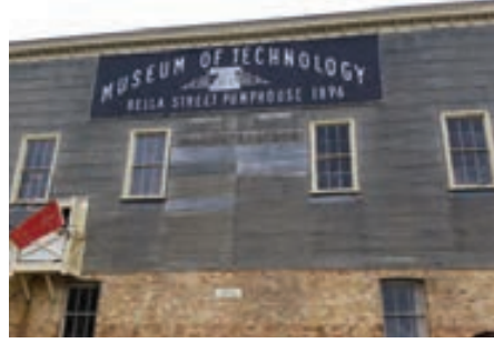
Bay of Plenty: Bella Street Pumphouse exterior.
