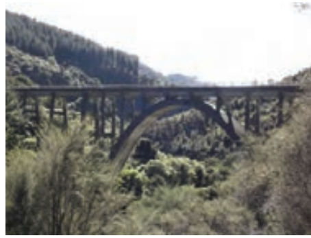
Gisborne: Kopuawhara Viaduct which had to be traversed to get to the Memorial Monument.
