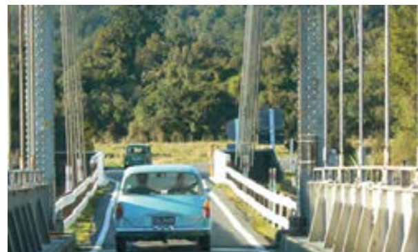
▲ Central Otago: Karangarua Bridge.
