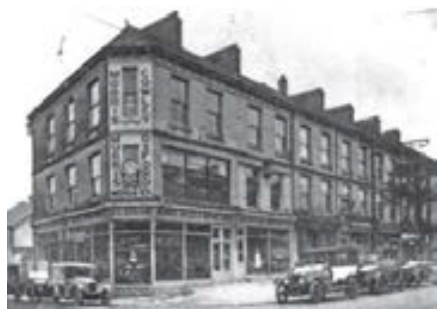
▲ A view of the Barton Motor Company's showroom at 54 Mutley Plain, Plymouth. A typical Morris Dealer of the 1920s.
